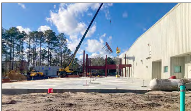
Phase 2. Completion of flooring and framing commences. Museum Photo.
